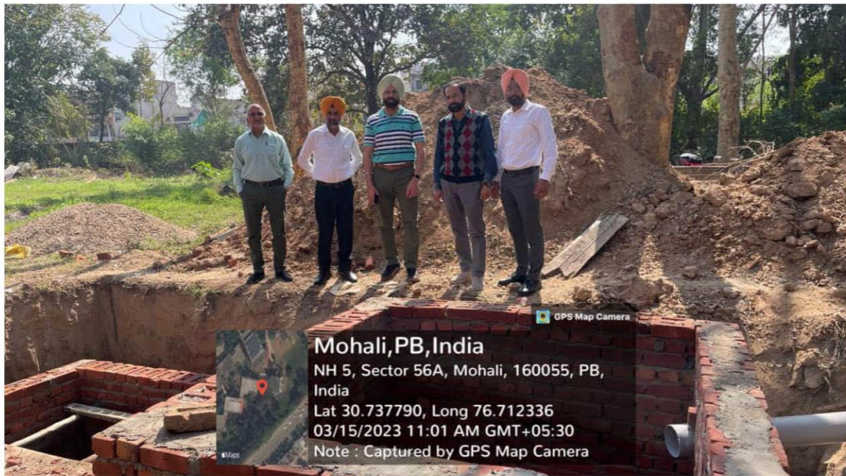
(Rainwater Harvesting System being constructed)
